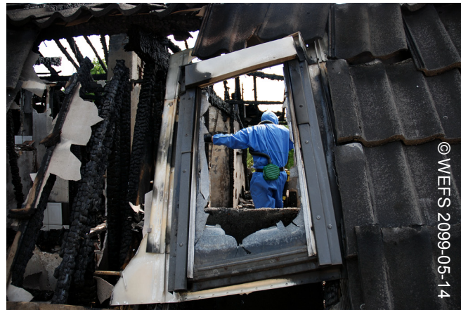
Asbestos removal work after a fire
